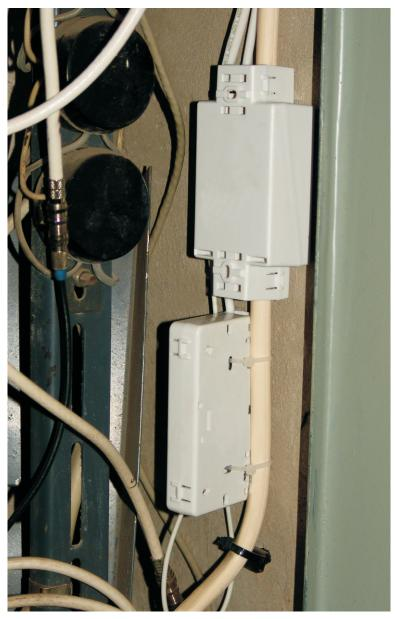
You can put FOS-18 either in distribution cabinet (switchboard) next to FOS-16 or elsewhere where you can make fiber connections through mechanical splice holder. At each splice holder is possible to connect up to two cables. Combining both products you can make quick and price-performance FTTH solution – at least one optical fiber for each subscriber.
