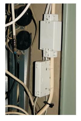
When installation complete, put the optical cable with fixed distributor FOS-16 to distribution cabinet (switchboard).
