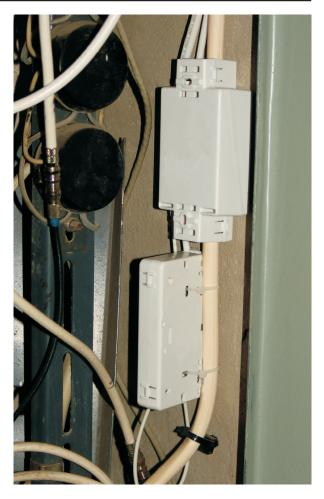
Distributor with cable strips are fixated with 10 mm or 15 mm thick optical cable and are covers partition. It is possible to lead out up to four fibers in every direction, up or down. Outgoing fibers are fixated with 5 mm plastic cover tubes. Plastic cover tubes are fixated in the distributor with cage washers which ensures strong fixation.
