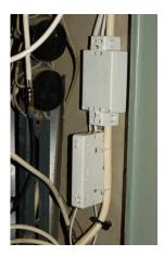
If You prefer mechanical splicing, FOS-16 & FOS-18 can be Your choice. FOS-16 is fiber optic breakout box, mounted on riser cable and provided for distributing up to four outgoing fibers. If it is necessary to extend fibers, there can be used mechanical splice in protective enclosure FOS-18 or FOS-23 also.
